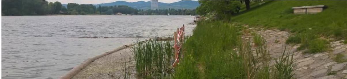
Revegetation of seawall
