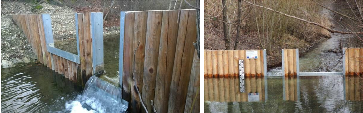
Measure weir Hebergraben
