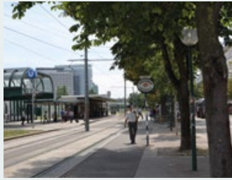
4.6.1 Cooling street-level and underground transport facilities
