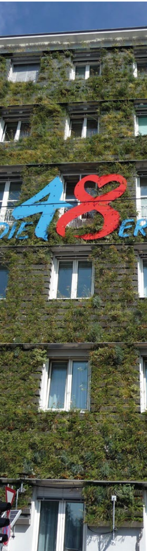
Good practice examples such as the MA 48 office building are important models for Vienna
