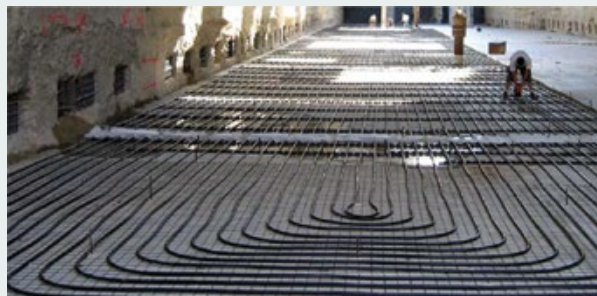
Geothermal collectors under the floor slab (source: civil engineers iC GesmbH)
