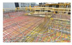
Hot or cold water is pumped through these pipes to heat or cool the building. © MA 20/A. Kromus
