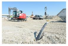
Step 5: Done: In the foreground, the top end of a borehole heat exchanger is visible - the other end is embedded 150 m deep in the ground.
