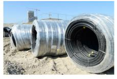
Step 2: Close up: the heat exchangers are delivered as coils of elastic pipe.
