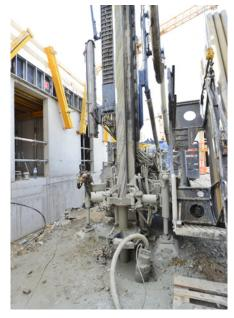
Renewable energy sources combined with concrete: A total of 30 borehole heat exchangers provide geothermal energy for efficient use in low-energy systems. © MA 20/A. Kromus
