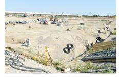
Step 1: The construction site in the summer of 2019. The overground portion of the underground line U2 is visible in the background. The two black coils in the foreground are the heat exchangers.
