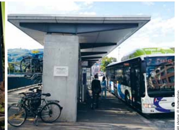
Combined bus stop and two storey bike parking facility in Olten
