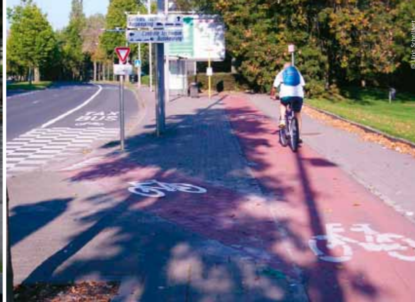
Bus/bike lane combined with cycle path on Avenue Paepsem: Cyclists can choose where to ride.
