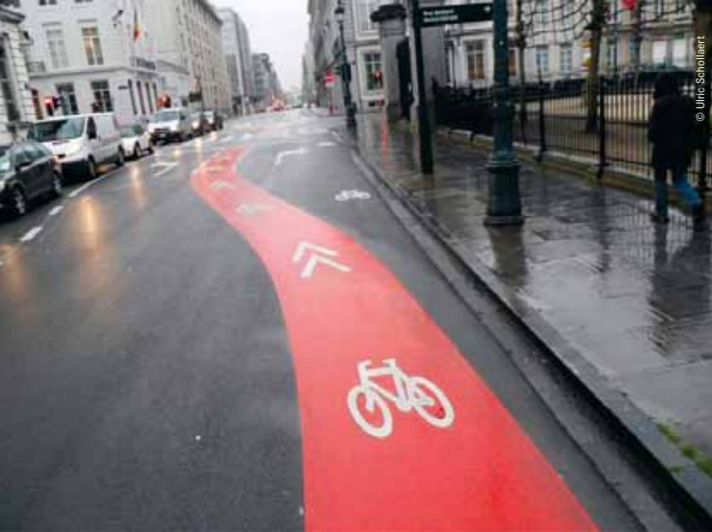
Junction on Rue de la Loi (cycle route). All cars must turn right or left – only cyclists are allowed straight on into the contraflow.
