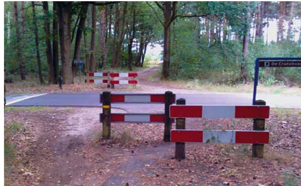
In the Netherlands, barriers placed to prevent moped drivers from the cycle paths seem to prevent cyclists from entering as well. (mistake No. 2)
