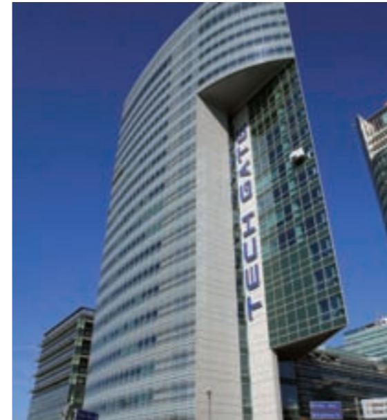
Tech Gate Vienna is the city’s top location for high-tech developments, offering all tenants an ideal platform to strengthen collaborations and informal contacts, which contributes to the dynamization of the technology and knowledge transfer process.
