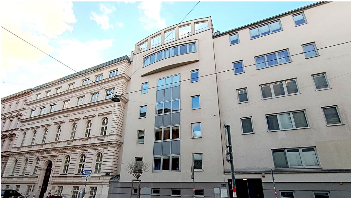
Figure 42: The residential buildings at Castellezgasse 35–37 © Schöberl & Pöll GmbH
